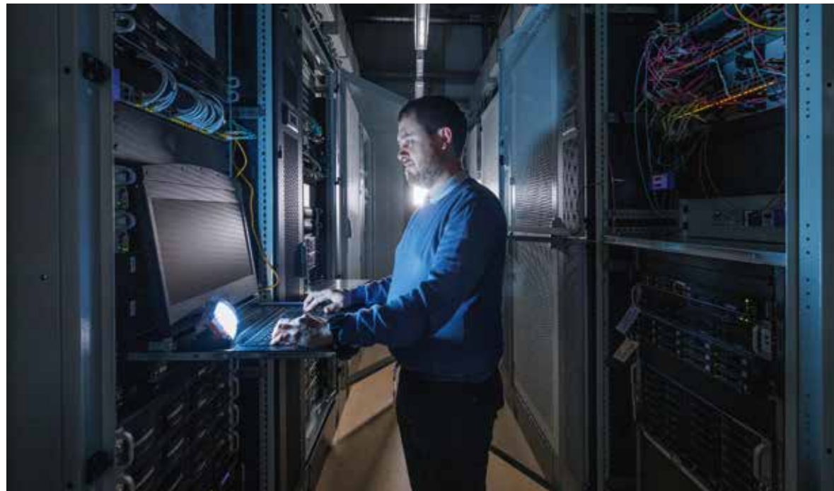
Login nodes, compute nodes, server nodes and storage nodes, all mounted in 19" racks and housed at the University of Vienna Biology Building (UBB). Credit: Joseph Krpelan
